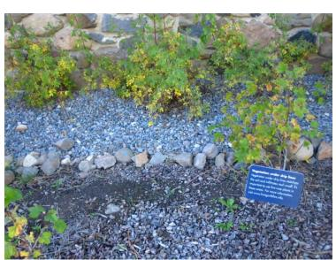
Vegetation under drip lines infiltrates roof runoff
