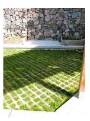
A rock gabion wall on the perimeter of the property extends 3-4 feet below the ground. The rocks in the gabions filter subsurface flows. Permeable pavers cover the restaurant's patio area.
