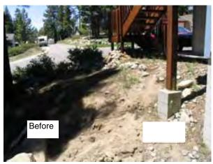
Above: Before Below: After This landscape project included slope stabilization as well as armoring below the dripline and beneath the deck.
