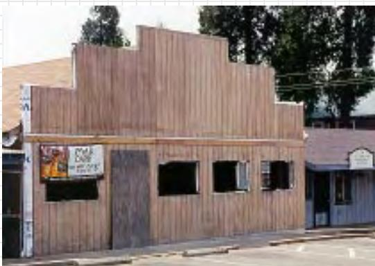
*The use of plywood panels without battens is inappropriate.*
