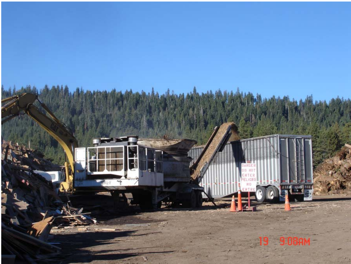
Loading Biomass in a truck for transport to energy facilities
